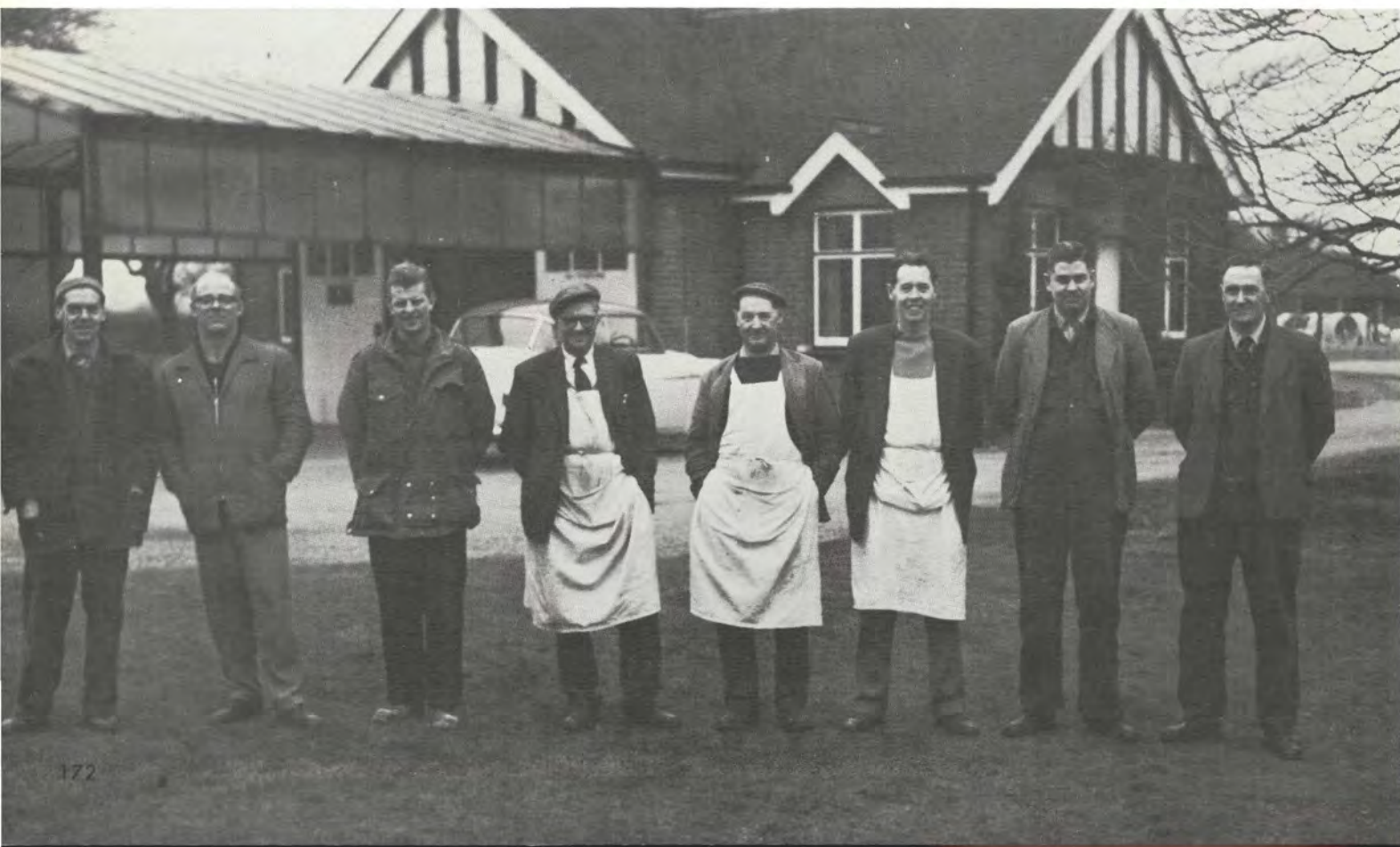
Construction Crew: (left to right) Philip Wagner, Herbert (Bert) Chadd, James Feld, Bricklayers; Wallace Burnett, William Marlborough, Peter Marlborough, Carpenters; Derek Wright, Electrician; Donald Akam, Plumber.
